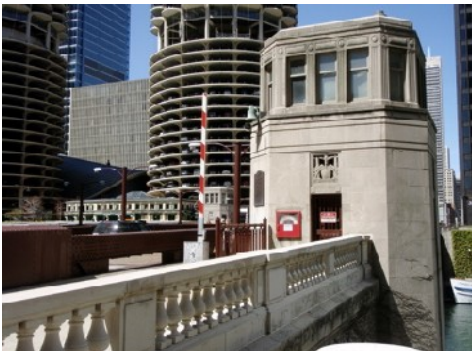
3. NORTH STATE ST. BRIDGE (BATAAN CORREGIDOR MEMORIAL BRIDGE) (1949)
